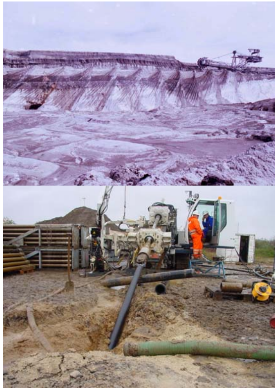
Figure 4. Mine section dewatered by HDD-well and drill rig at open pit mine „Vereinigtes Schleenhain“
